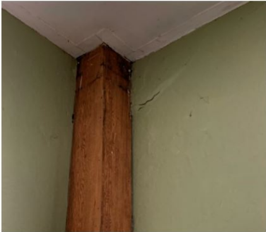
PHOTO #8: At various points in the facility, there is water/moisture damage leading to cracking in the plaster walls.
